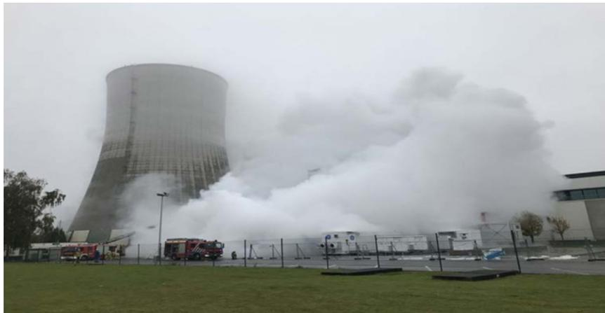
An Engie Ineo lithium-ion utility-grid BESS experienced a large fire in 2017 as seen in Figure 22. The incident occurred at the test facility during commissioning. The 6 MW facility was to be used for grid balancing, and was the first time such a facility was to be used for that purpose in Belgium. The damage to the BESS was considered a total loss.<sup>98</sup>
